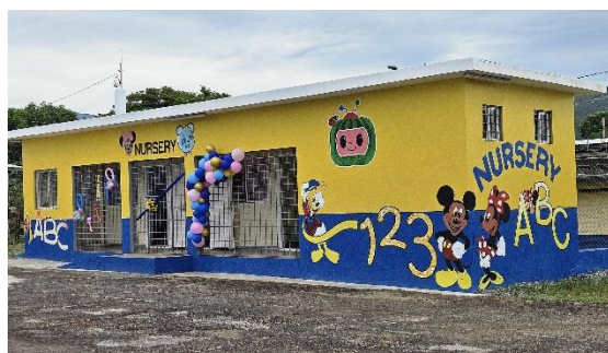
Newly constructed nursery at the South Camp Adult Correctional Centre in Kingston.
