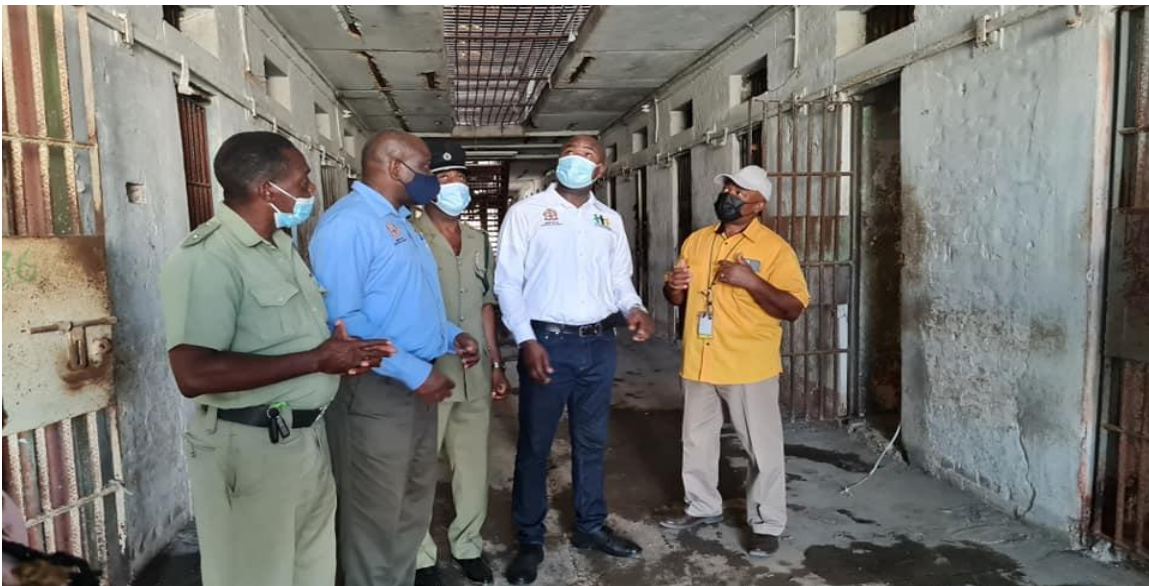
Infrastructural Inspection of Cell Blocks within the Correctional Centre
